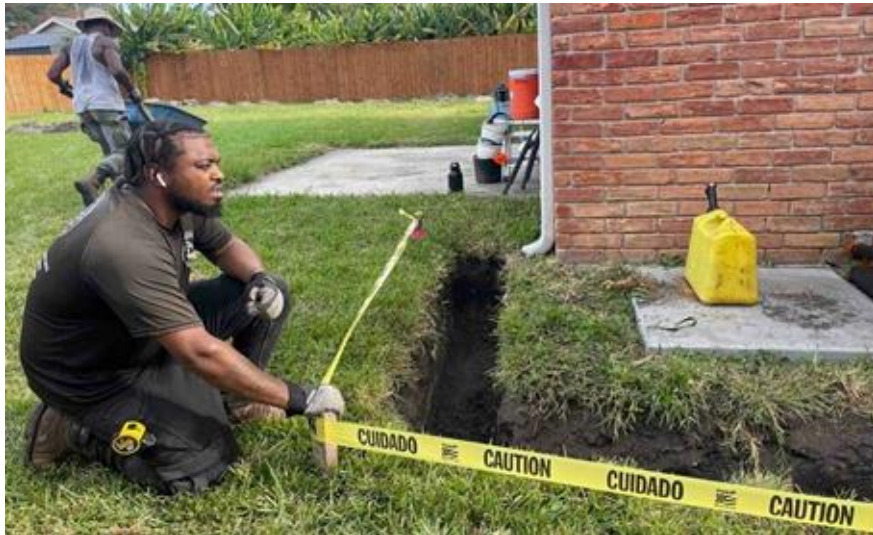
French Drain Installation on Jahnke Road
