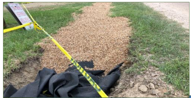
Figure 12 - Stormwater drainage being installed. Image credit: EPR PC
