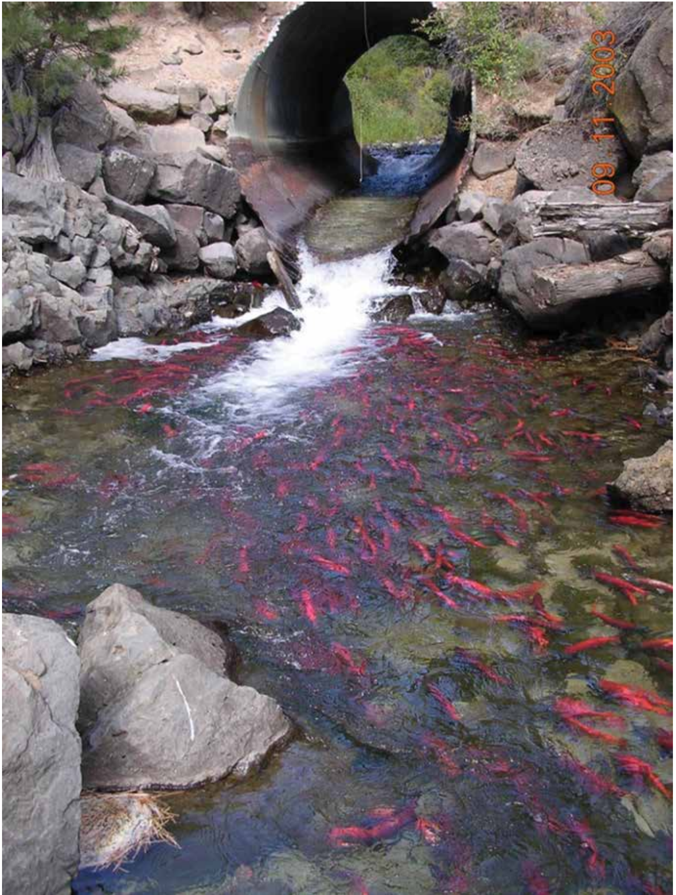
Plate 1. Climate change may exacerbate many habitat fragmentation issues like this blockage of a kokanee salmon migration by low summer flows at a poorly fit road culvert. Photo credit: Clayton Nalder.
